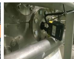
NH3 sensor installed in stack
